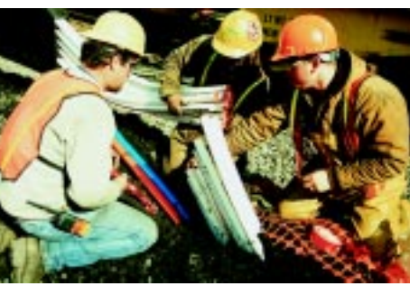
Crew prepping tie-in for multiple duct installation.
