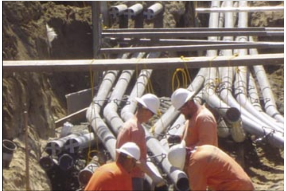
H&M crew installing 69 kV duct bank.
