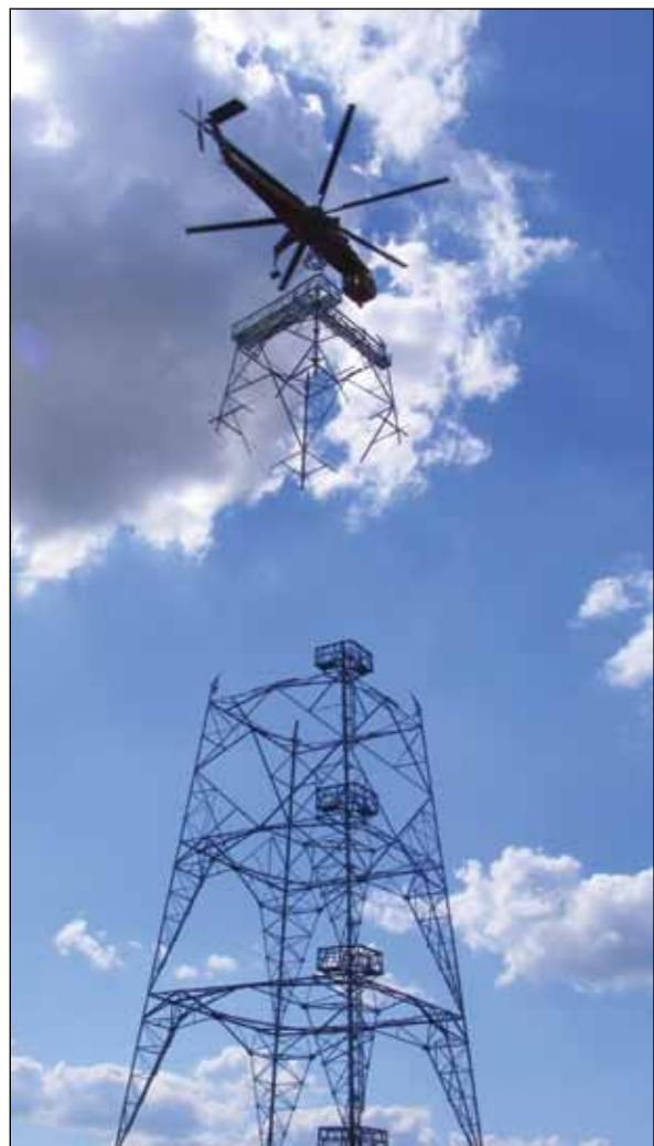
*Water component of the Vectren Gibson-Brown-Reid 345 kV Transmission Line Project involved utilizing a barge to help construct a 265-foot tall lattice tower on an island in the Ohio River (base under construction, left); Air components of the project included extensive use of choppers (a lattice tower is capped via helicopter, top).*
