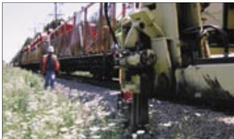
*The H&M Railroad Mounted Cable Plow installs and buries cable to a depth of up to six feet. A backhoe following the train completes installation by leveling any displaced stone on or near the track bed (below).*
