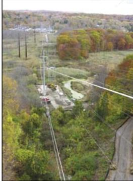
structures because of constraints such as terrain and the fact that the line traverses residential neighborhoods." Crews had as little as five feet clearance between the existing lattice tower and the conductors, so NU reconfigured their grid to maintain full service while the conductors were de-energized.
