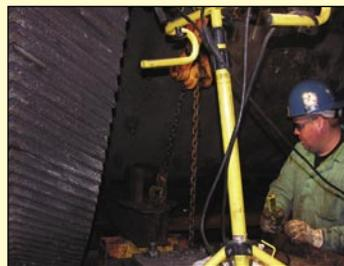
Bobby Nelms, the H&M Industrial Group jacked up the 1,100-ton unit, rigged, and lowered the old bearing assembly (8,000 lbs) to the ground, raised the new bearing, and rigged it into place. The job required some difficult manual rigging. H&M was given an award for quick response and outstanding service in returning the plant to full capabilities. Greg Class, Director,
