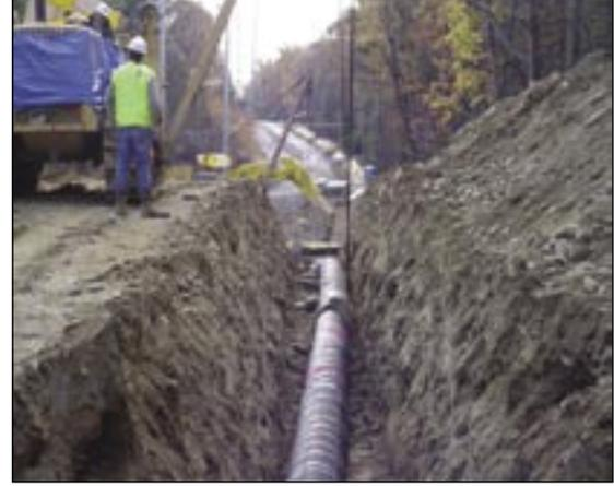
*H&M Pipeline Division, replacing old 14-inch pipe with new 20-inch pipe in Pike County in Pennsylvania's Pocono Mountains for Columbia Gas Transmission. Rugged conditions warrant a double rock-shield wrap.*
