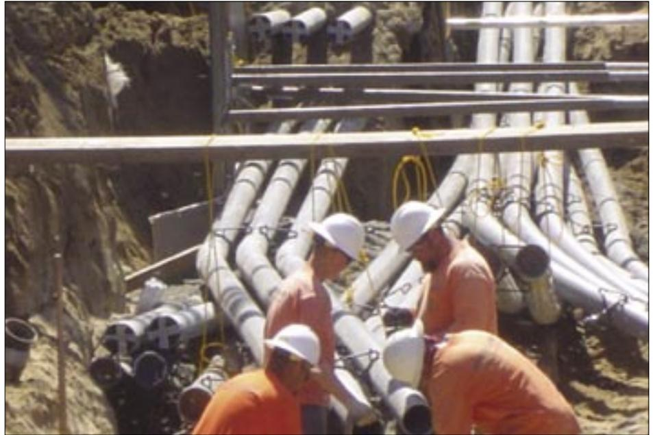
H&M crew installing 69 kV duct bank.
